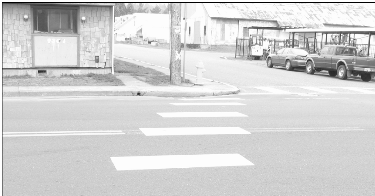
Figure 5 Crosswalk without Accessible Curb Ramp
